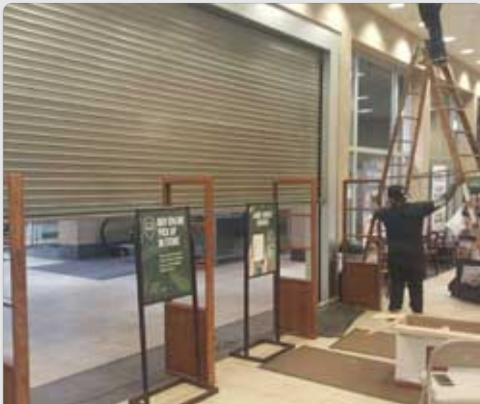
Commercial Gate Installation
